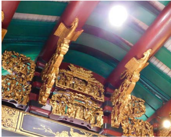
Figure 17a Corbel brackets featuring two distinct designs of phoenixes, 2021.
