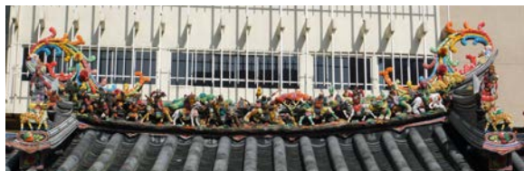
Figure 3a The gateway roofscape featuring the Baxian.
